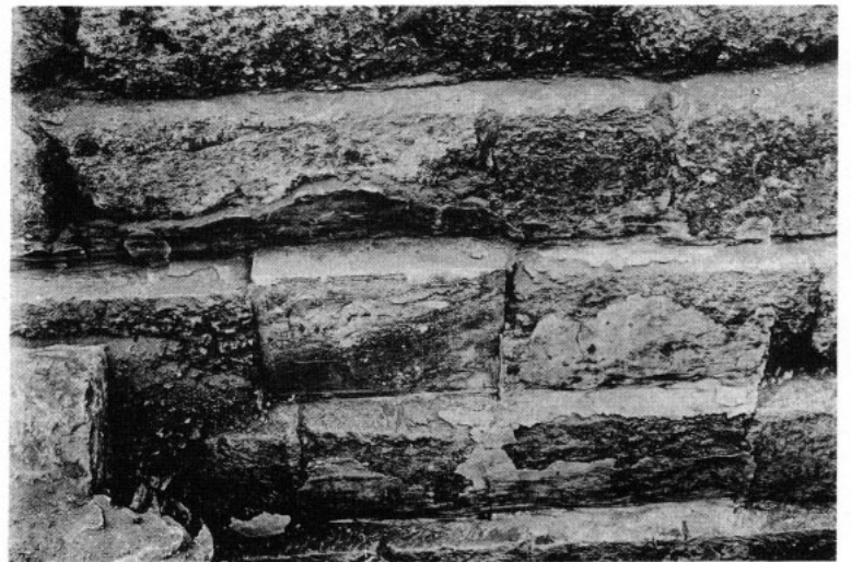
f. G 1223, Slab-stela in place in retaining wall of core: 1904-5.
