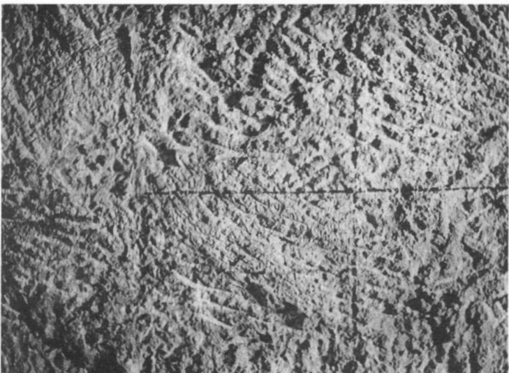
e. G 1203 A, Red construction lines and chisel marks on ceiling: 1905.
