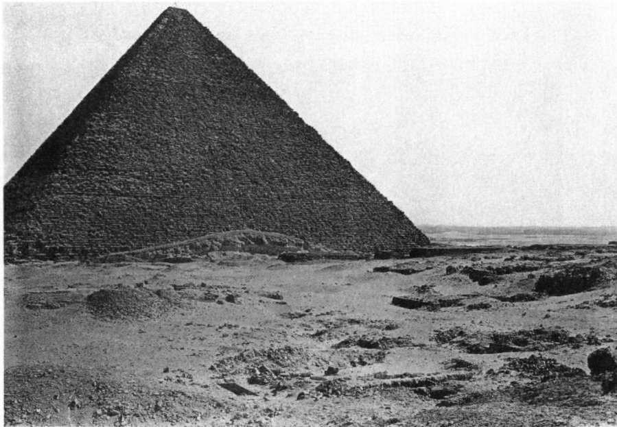
c. Cem. G 2100 before excavation, looking ESE from G 2000: 1905.
