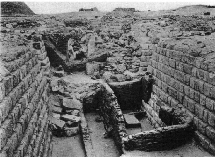
e. G 1235, Exterior c.b. chapel of type (1 a), looking SSW: 1905.
