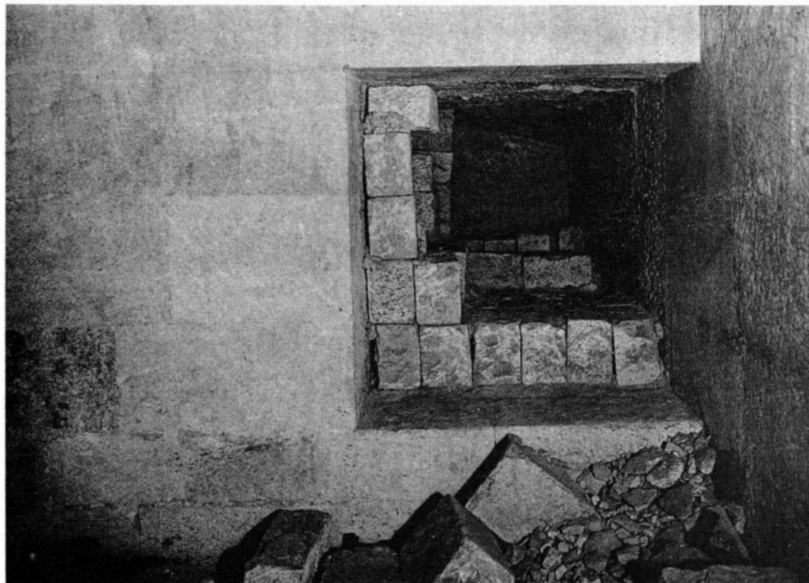
c. G 2100 A, North wall of chamber and blocking in passage: 1905-6.
