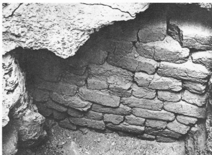
d. G 1233 annex, Shaft looking south, interior c.b. blocking of passage: 1905.
