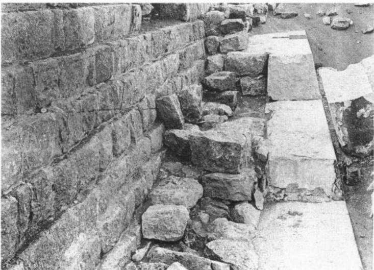
e. G 2130, Casing and core, middle of east face, looking north.
