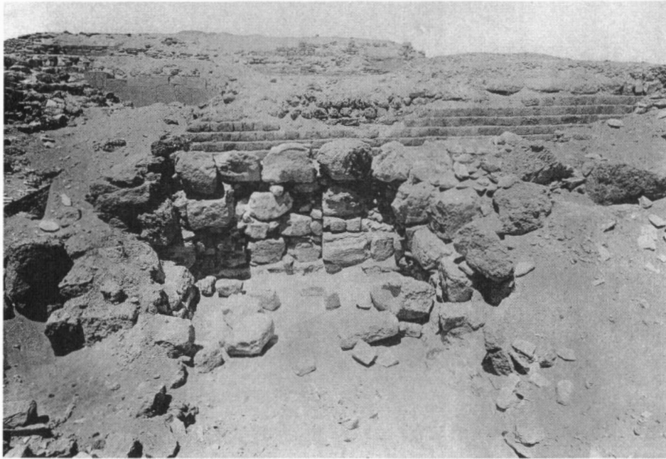
a. G 2210, South end, looking west; stepped core, massive enlargement, and chapel recess: 1935.
