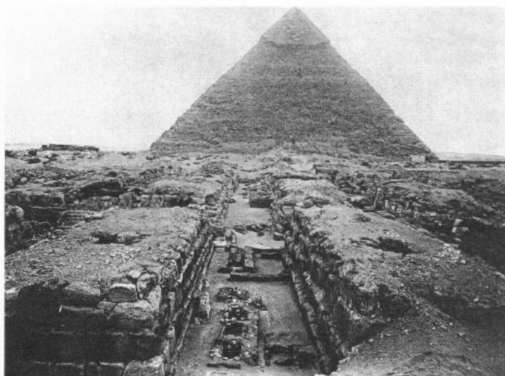
d. G 4540, Street between G 4540 and 4560 showing chapel, looking south: 1914.
