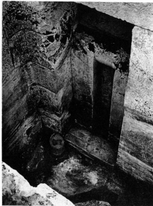
c. G 4240, Chapel, ka -door, looking down to west: 1914.
