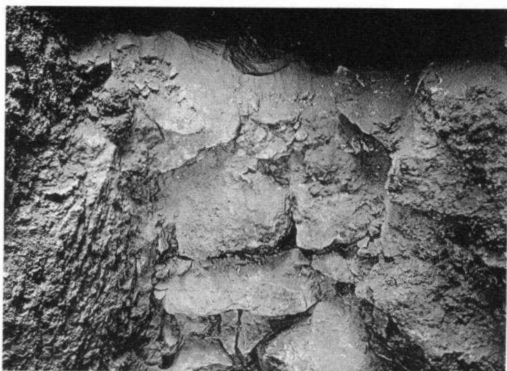
a. G 4620 A, Blocking of type II c (2) penetrated by thieves, looking south: 1914.
