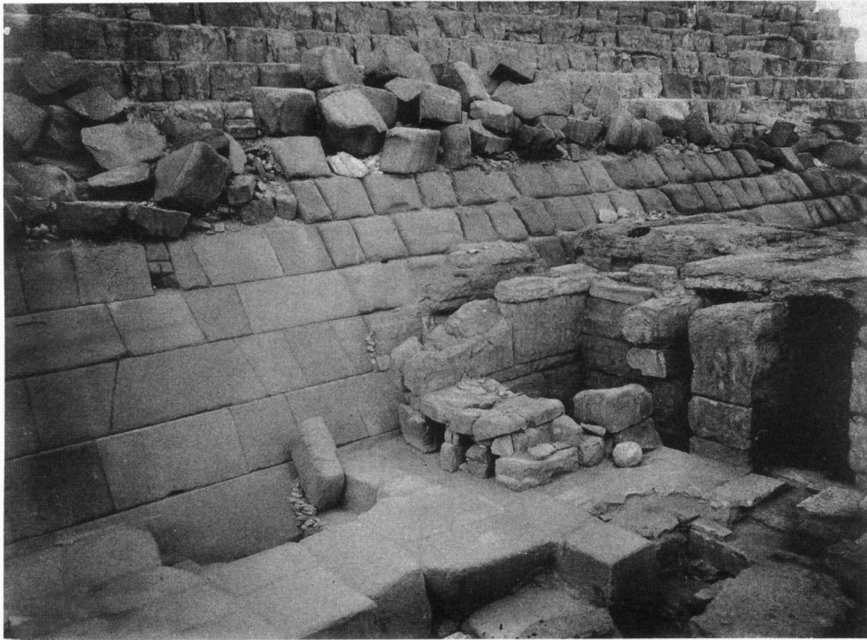
a. M. P. T., room (29), granite pavement and granite casing of pyramid, looking northwest, October 20, 1923.
