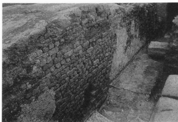
b. M. P. T., northern corridor (13), south wall, crude-brick casing partly stripped of plaster, looking down to W. S. W., October, 1923.
