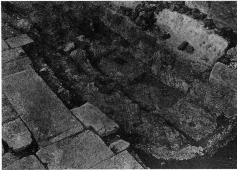
c. M. P. T., court (5), east wall, south part, emplacements for granite casing, looking down to N. E., June, 1907.
