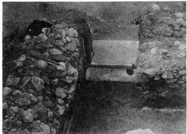
f. M. P. T., room (36), doorway, looking down north, April 12, 1907.
