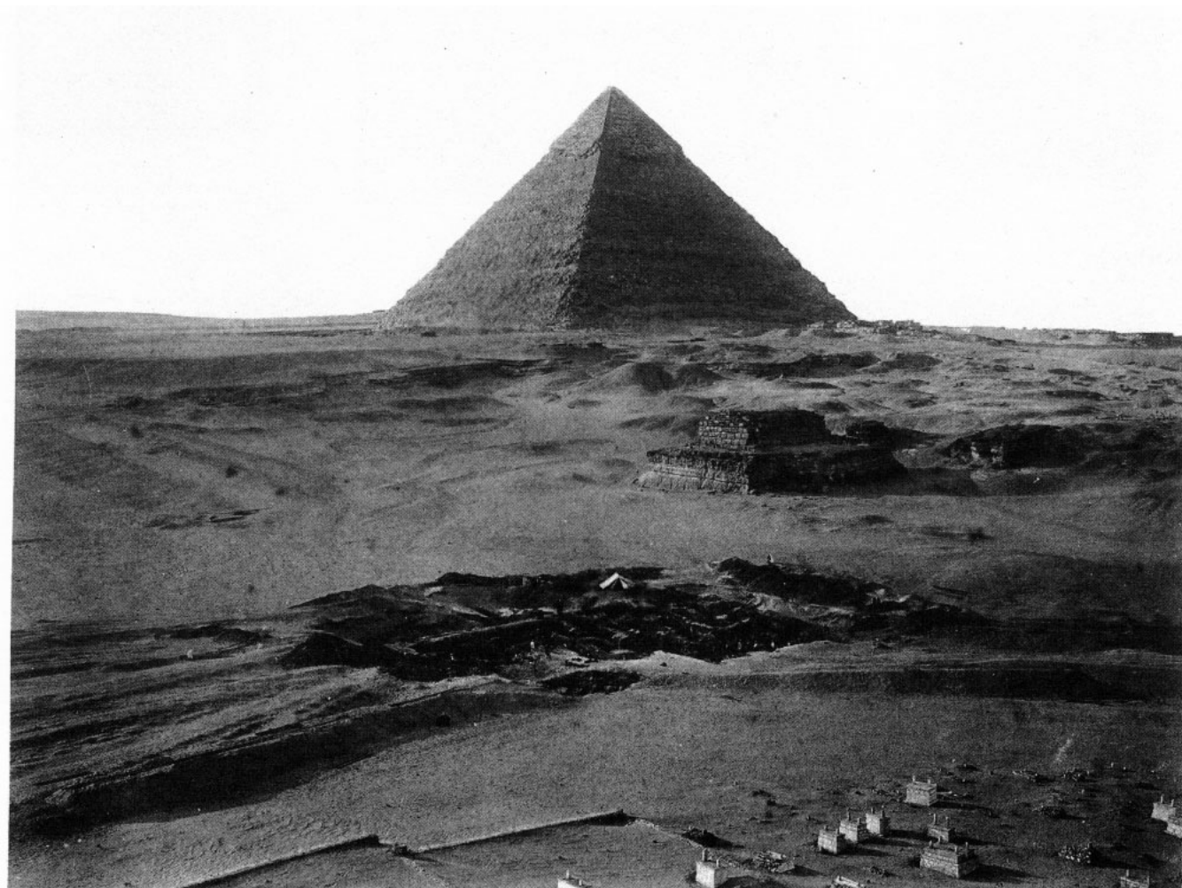
b. Micerinus Valley Temple, after excavation of western part of temple, looking northwest, February 9, 1910.
