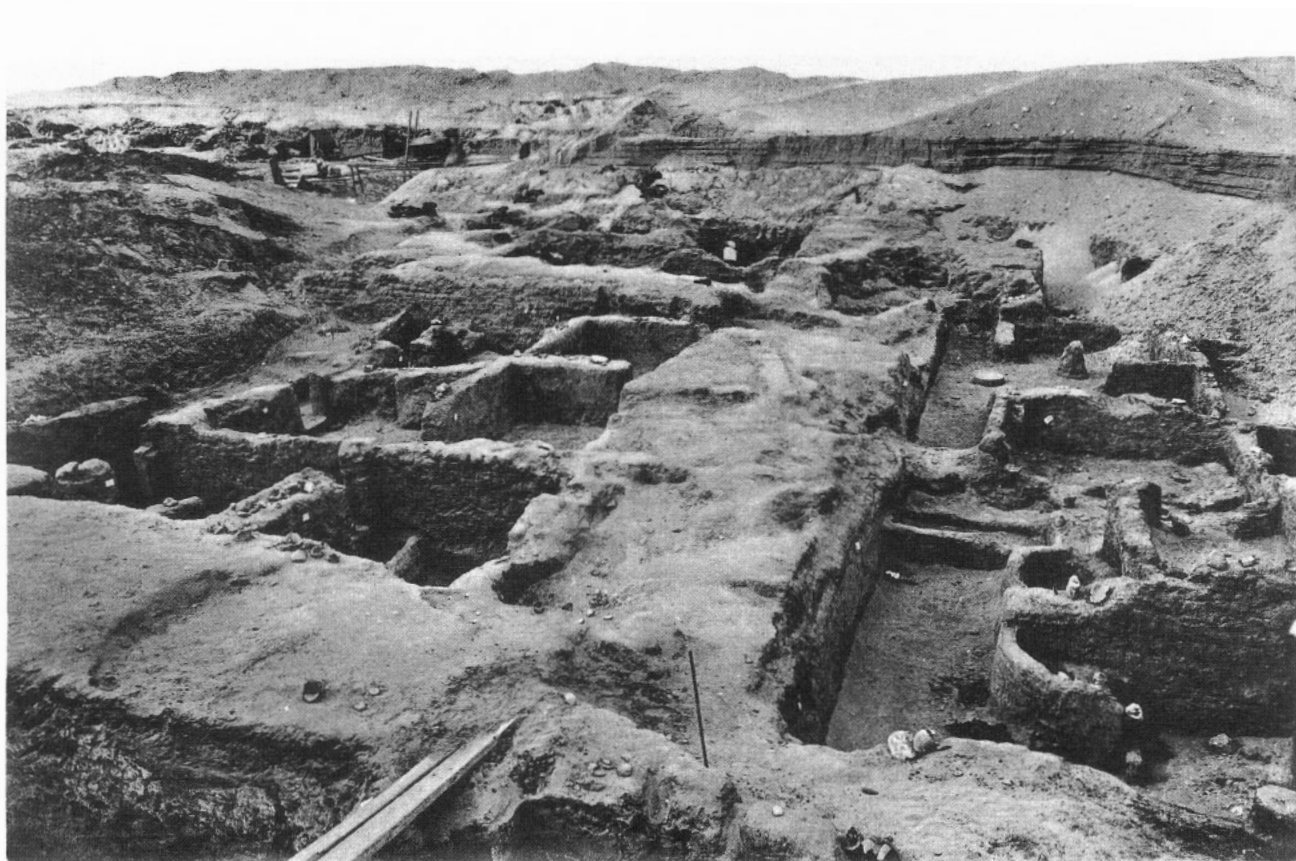
a. Mycerinus Valley Temple, vestibule and houses east of temple, before removing wall of vestibule of Second Temple, looking N. N. W., March 15, 1910.
