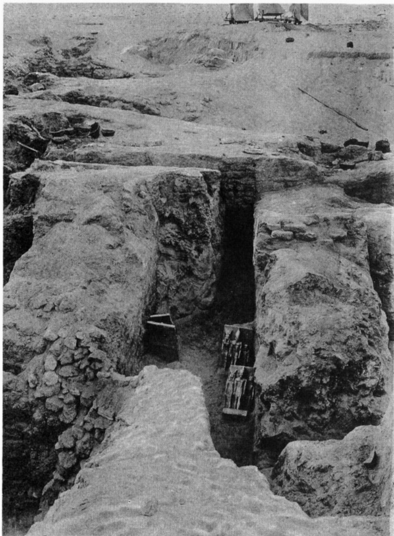
a. M. V. T., corridor (4), the four triads as found, looking north, July 10, 1908.
