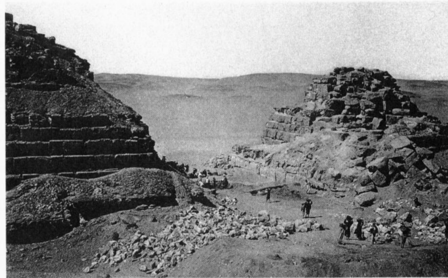
b. M. Q. T. Small pyramid III-c, surface of decay, beginning of excavation of debris of decay in portico, looking down to southwest, July, 1924.
